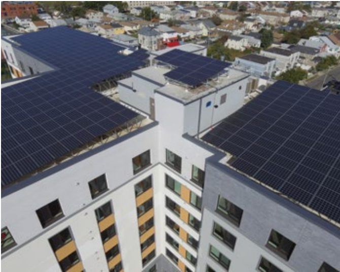
A 133 kWh solar array on the roof supplies nearly all of building's energy needs.
