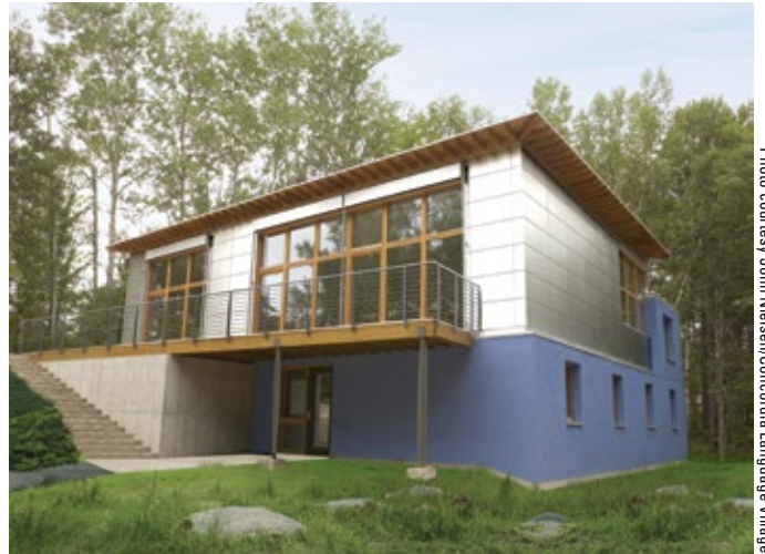
The first building in North America to be certified by Germany's Passivhaus Institute is the 5,000 sq. ft. Waldsee BioHaus in Bemidji, Minnesota. It used Amvic ICFs for all exterior walls.
